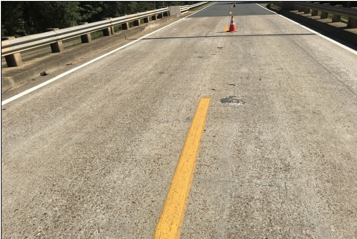
Span 48 looking ahead @ deck overview with some minor spalls.
