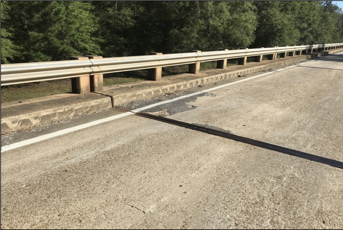
Span 2 Lt. Side from bent 2 ahead there is a patched spall in gutter line approx. (2 1/2' x 6'). This is typical of spans 1 - 5.
