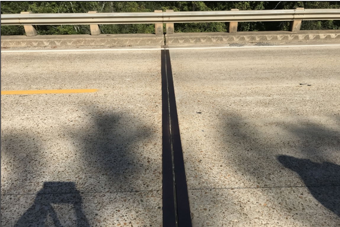
Bent 20 looking across @ joint repair, this joint is in good shape.
