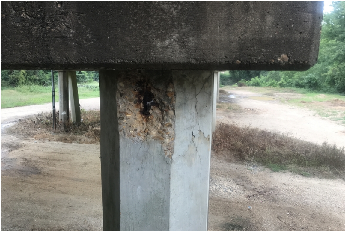
Bent 21 pile 4 spall with exposed rebar
