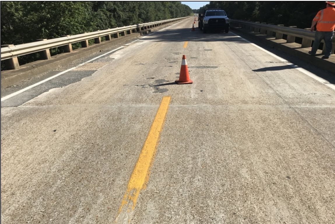
Span 26 looking ahead @ numerous deck spalls on entire span.
