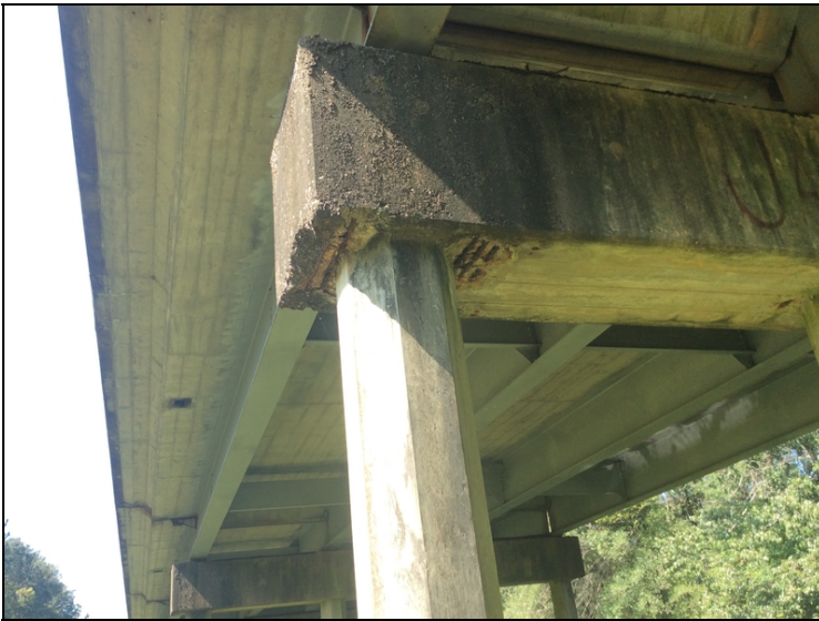
Bent 15, pier cap @ pile 4 has spalls both sides of the pile with significant section loss to exposed steel.
