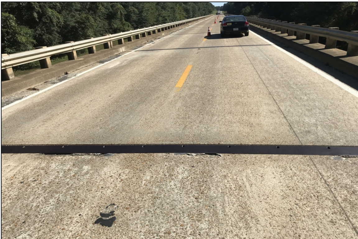
Span 28 looking ahead @ span 28. There is some minor spalling on the back side of joint between 28 & 29. There is also some deck spalls in Lt. gutterline.
