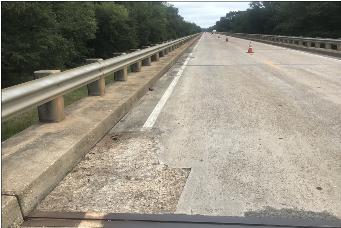
Spans 1-5, sb lane gutters have patches.
