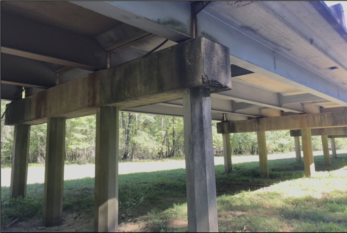
Bent 9 cap spalled right side
