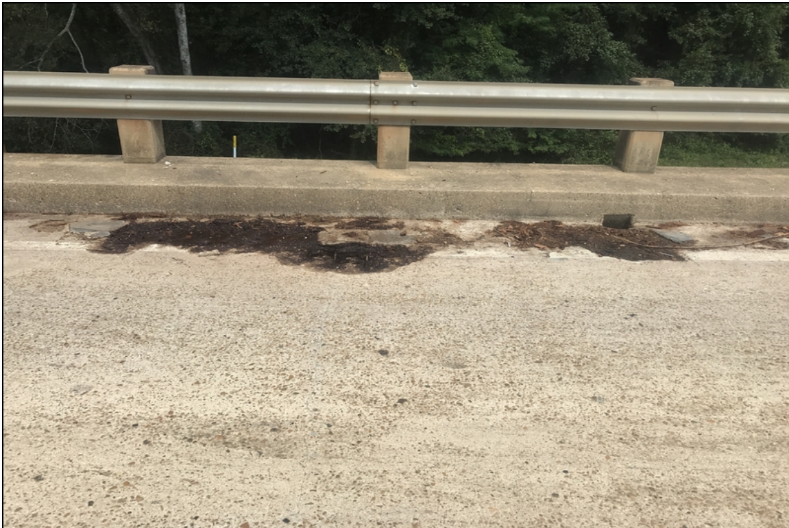
Span 28, sb lane spalled in gutter line.
