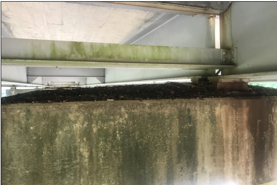
Bent 23 cap debris Also typical of bent 25
