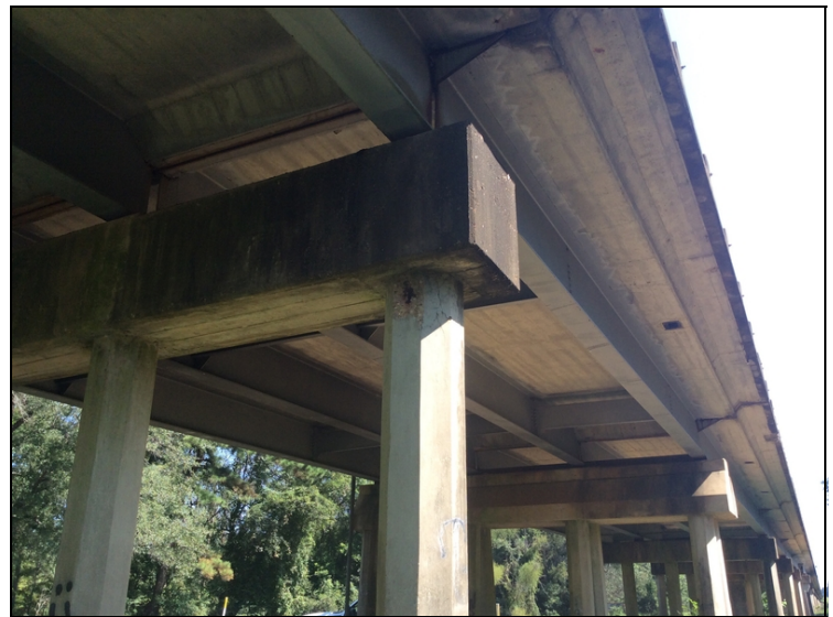
Bent 21, Pile 4 back has spall with exposed steel.
