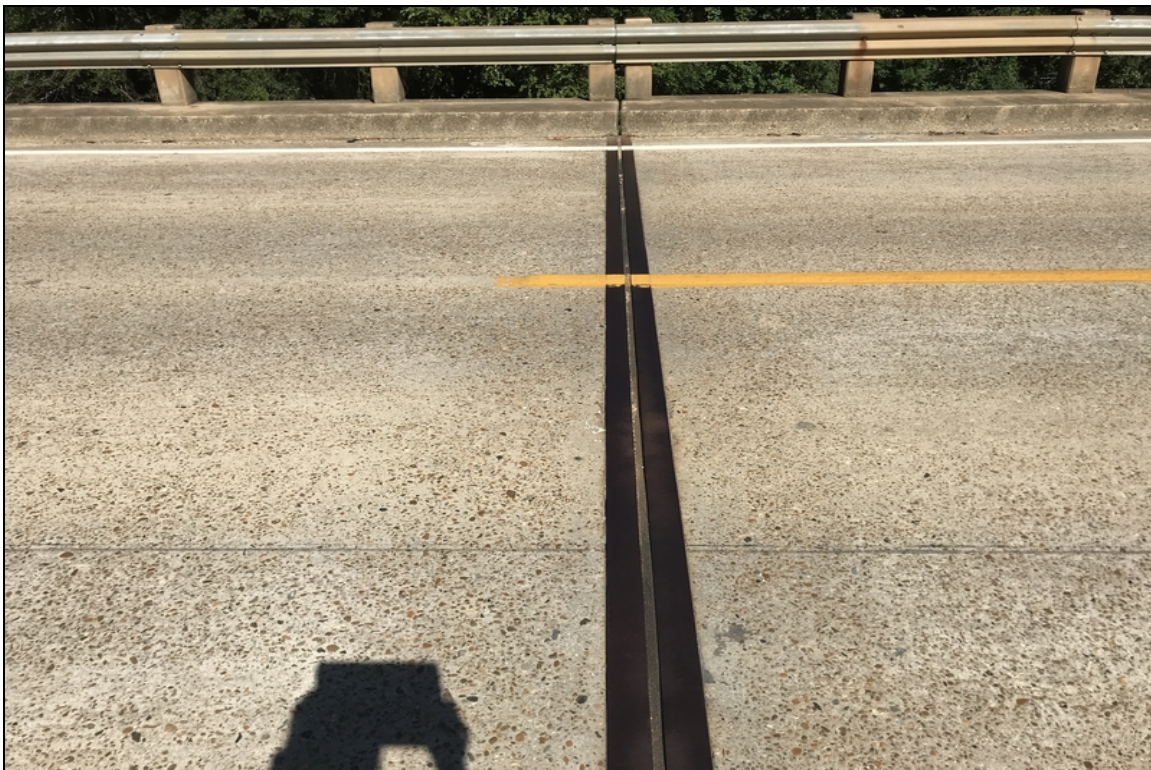
Bent 44 looking across @ joint repair.
