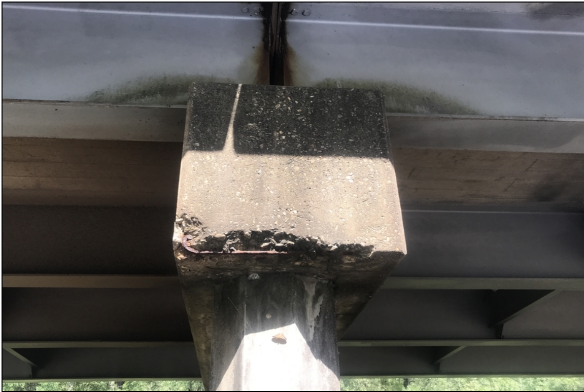
Bent 9, right end of cap spall with exposed rebar.
