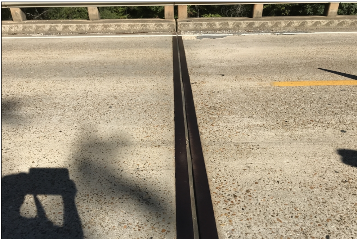
Bent 5 joint material has been repaired, typical of all joints.
