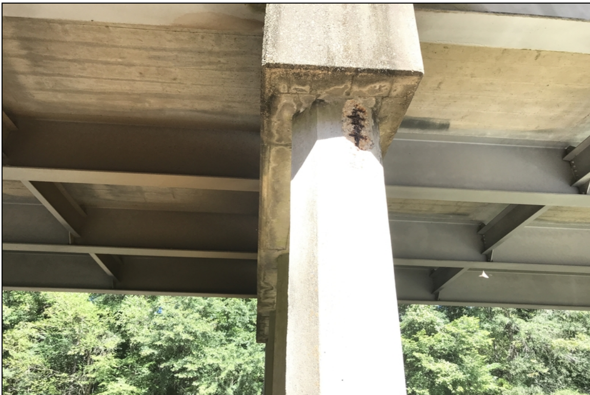
Bent 41 pile 4 spalled
