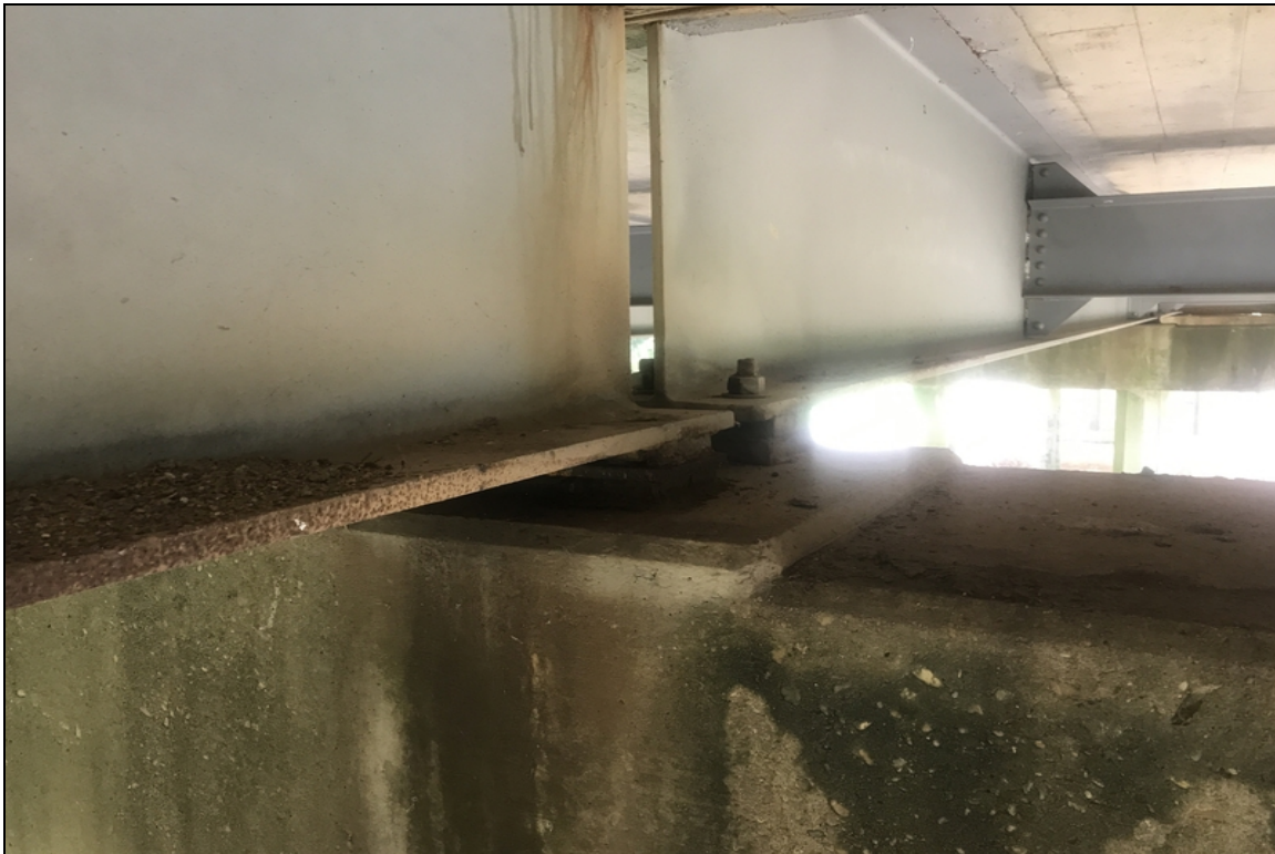
Bent 20 beam 3 bolt missing in bearing.
