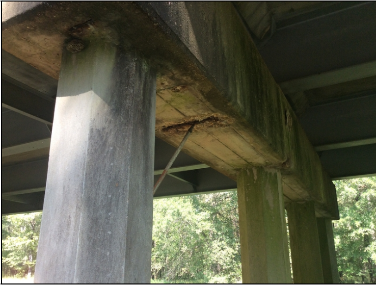
Bent 8 cap spalled with exposed rebar
