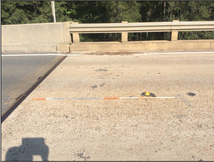
Deck spall, Span 1 2' ahead of BR begin, Lt. lane just outside the white line, is 7' long & 2' wide & about 2" deep at the deepest point.
