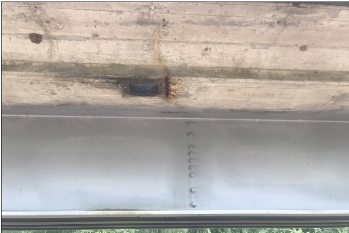
Span 23 drain hole
