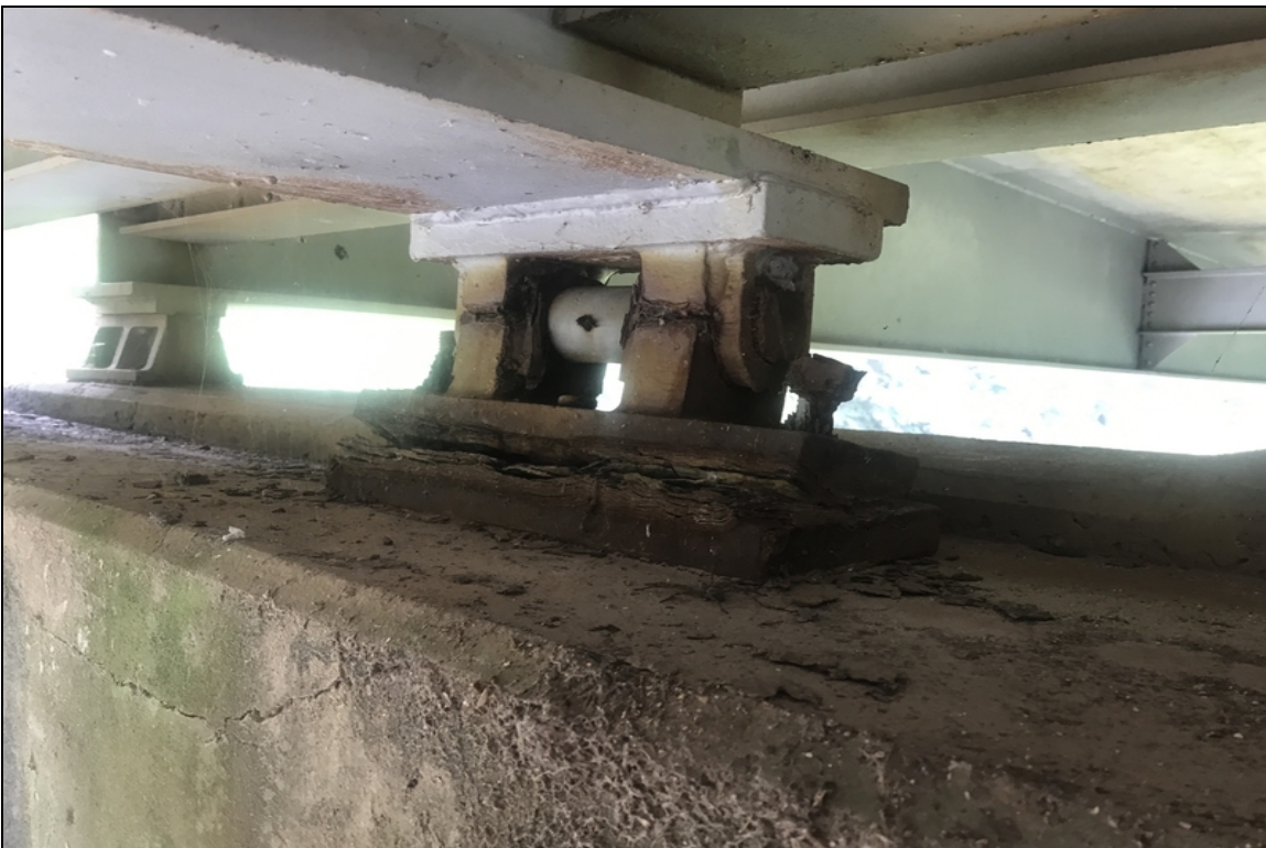
Beam2 bent27 bearing pack rust
