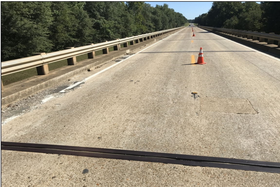
Span 36 looking ahead @ deck overview with some spalls mainly in Lt. Gutterline.
