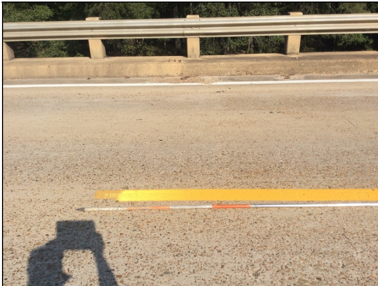
Deck spall, Span 1 Lt. lane 4' long x 2' wide x 1" deep about midspan.
