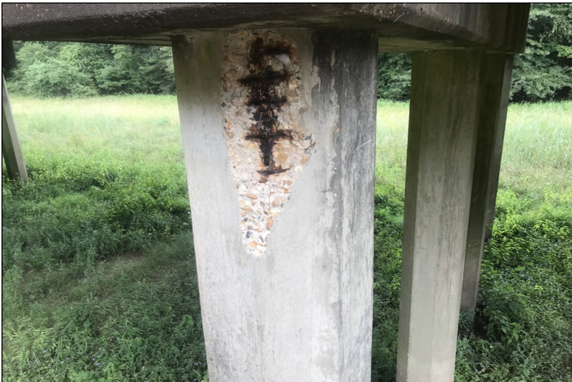
Bent41 pile 4 spall with exposed rebar
