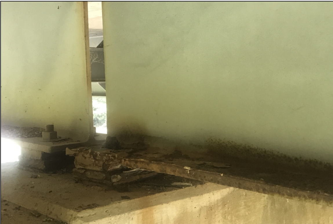
Bent 19, beam 2, typical of minor rust , with pack rust to bearing.
