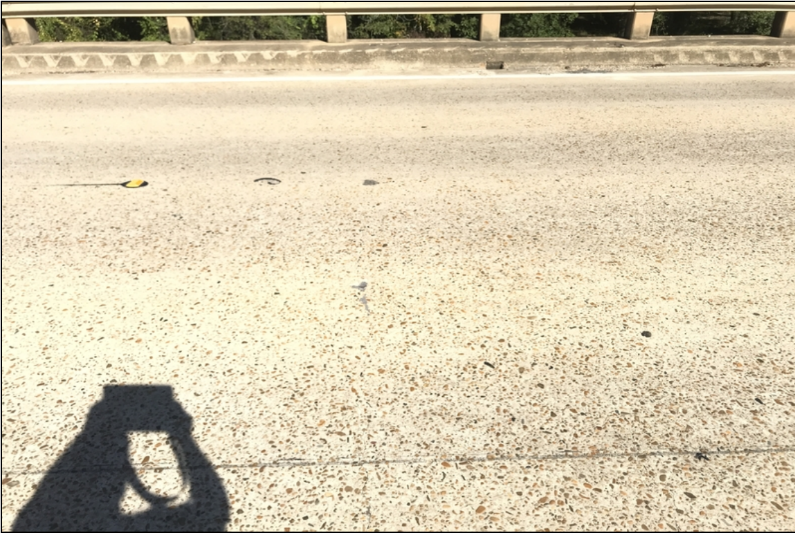
Span 21 looking across from Rt. to Lt. @ deck cracking, this is typical of numerous spans. There is also significant wear & abrasion to the spans.
