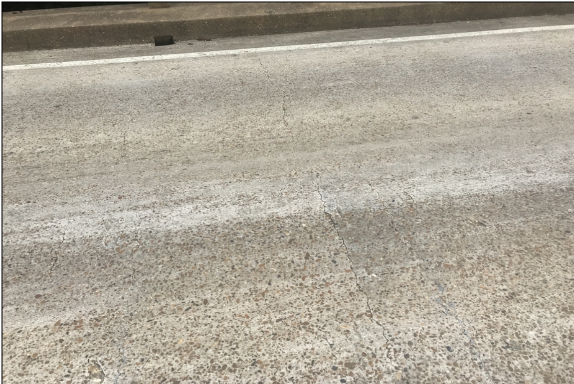
Span 8, moderate transverse cracks, max 0.040.
