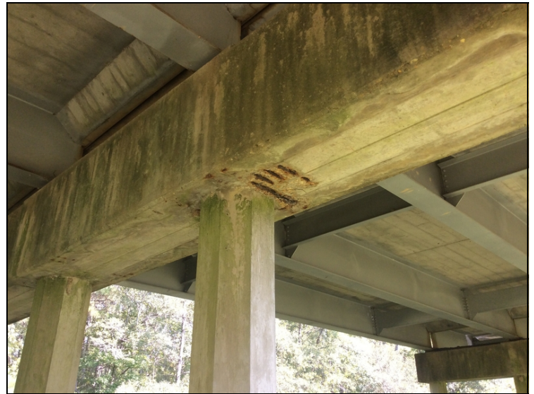
Bent 13 between piles 3 & 4, spall on the bottom of the pier cap with exposed steel with section loss.
