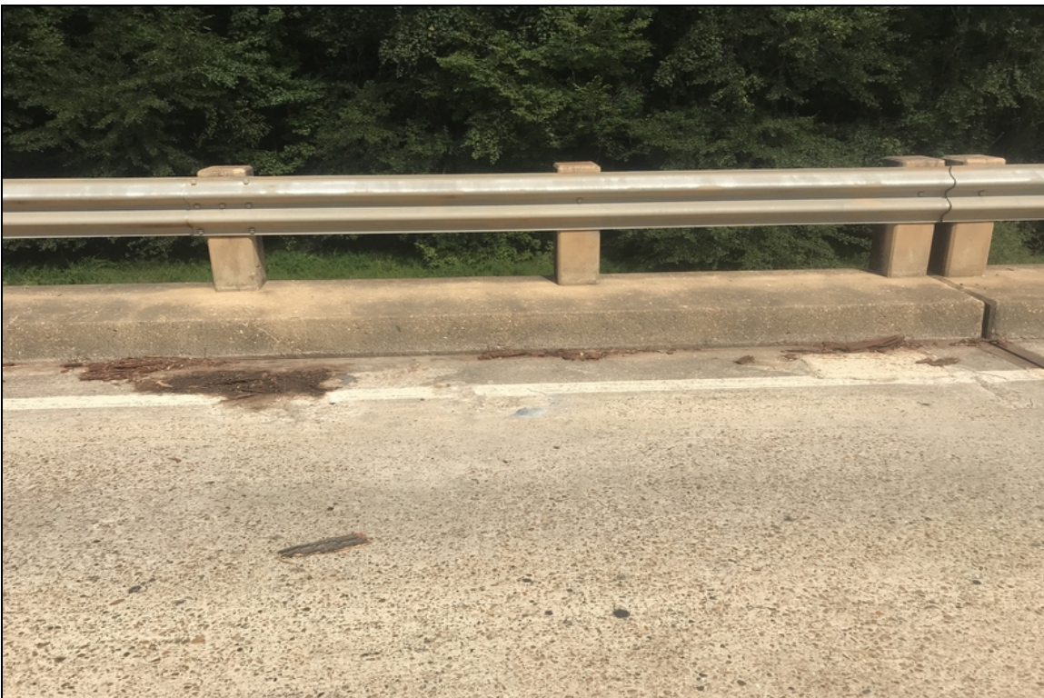
Span 41, deck spalls and patch.
