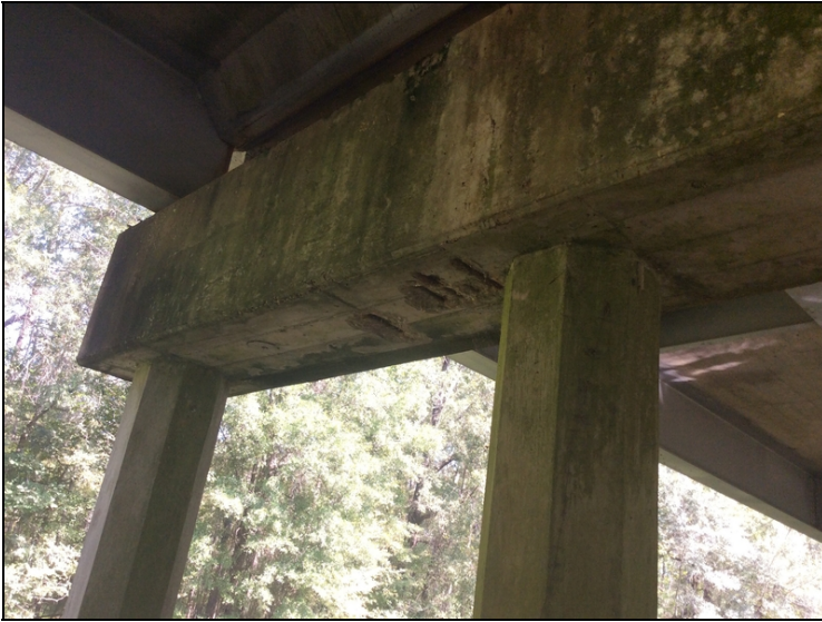
Bent 7 cap spall.
