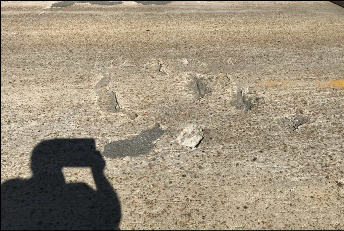
Span 23 @ C/L & 10' back of Bent 24 there is a spall with exposed rebar.
