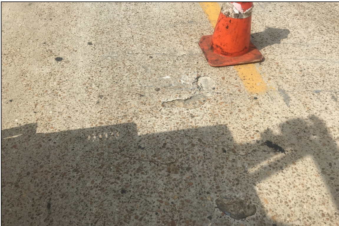
Span 48, spalls with transverse cracks.
