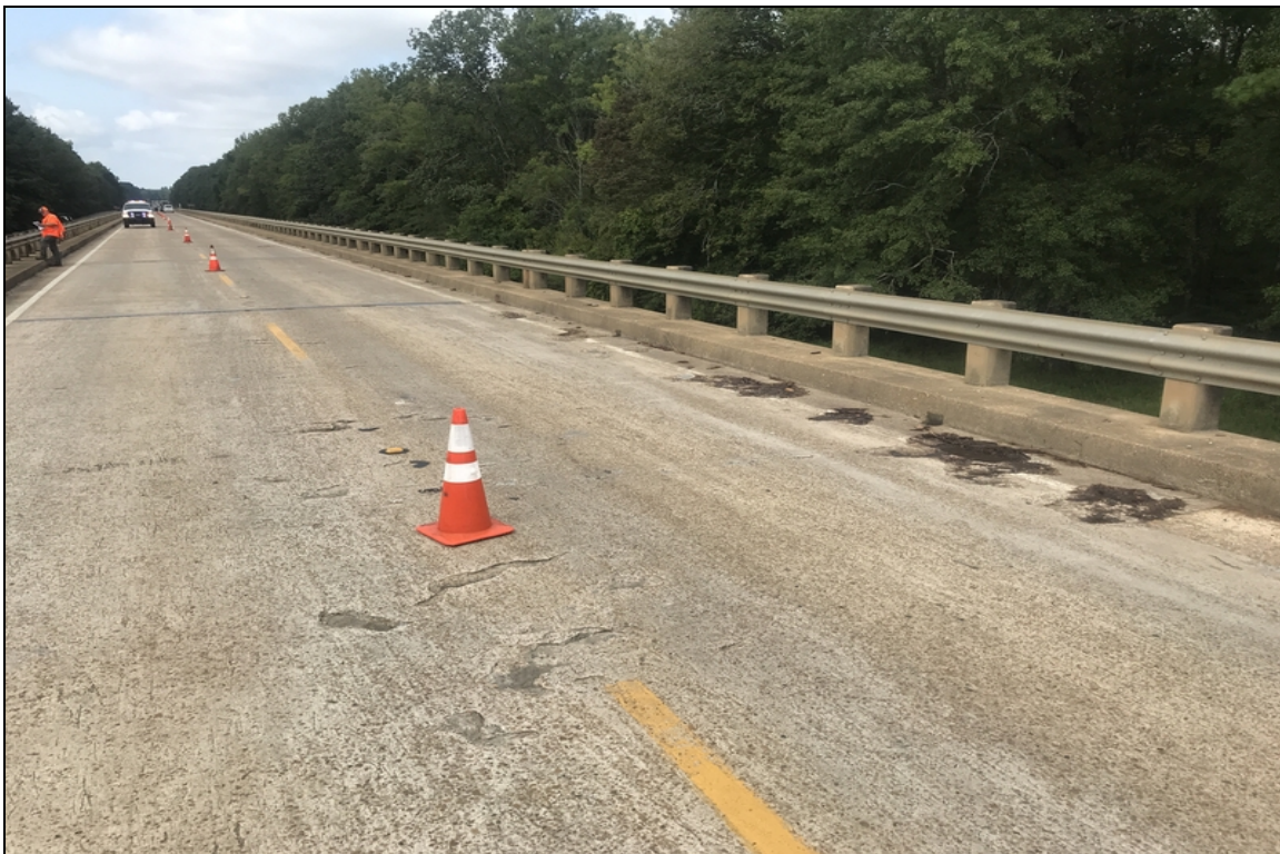
Deck overview span 23, spalls exposed rebar.
