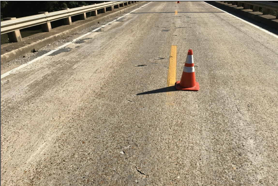
Span 23 looking ahead at deck overview with numerous spalls. There are several fairly large patched spalls in Lt. Gutterline & several smaller spalls Lt. & Rt. Of C/L. There are also numerous scaling & light spalls in the Rt. gutterline.
