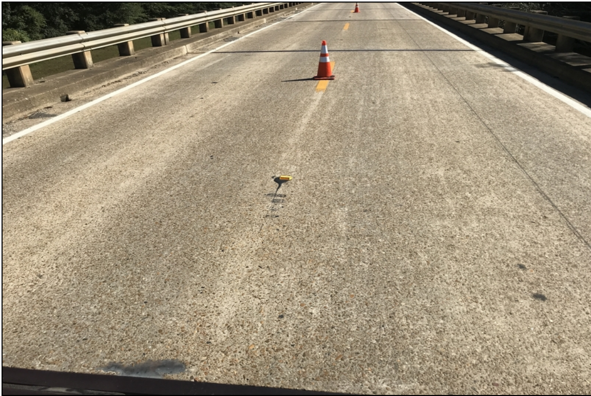
Span 34 looking ahead @ deck overview. There are some small spalls in Lt. gutterline.
