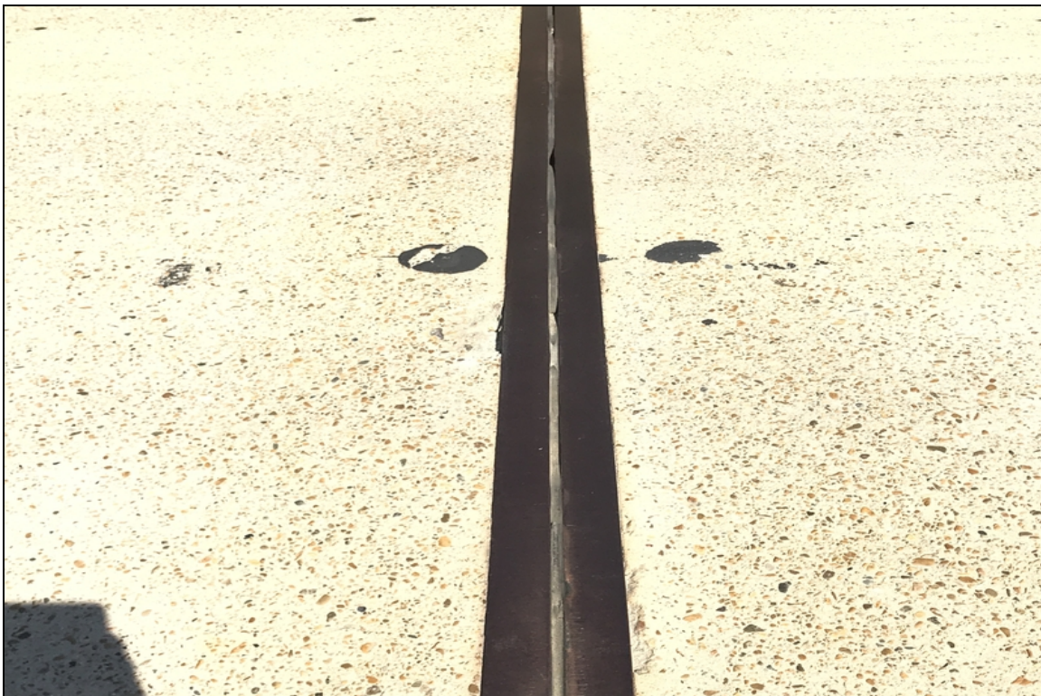
Bent 14 looking across from Rt. to Lt. @ joint material, there is some separation in the poured joint material from C/L Lt. in the SB lanes.
