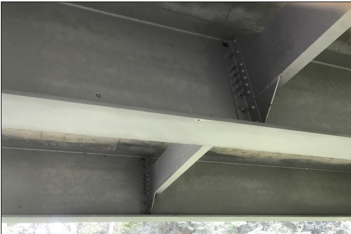
Span 27 missing bolts
