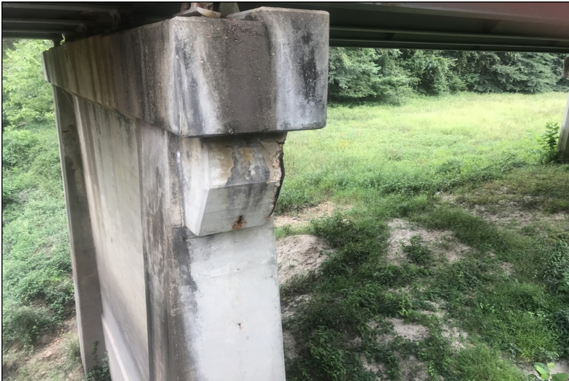
Pier 2 spall with exposed rebar right side end
