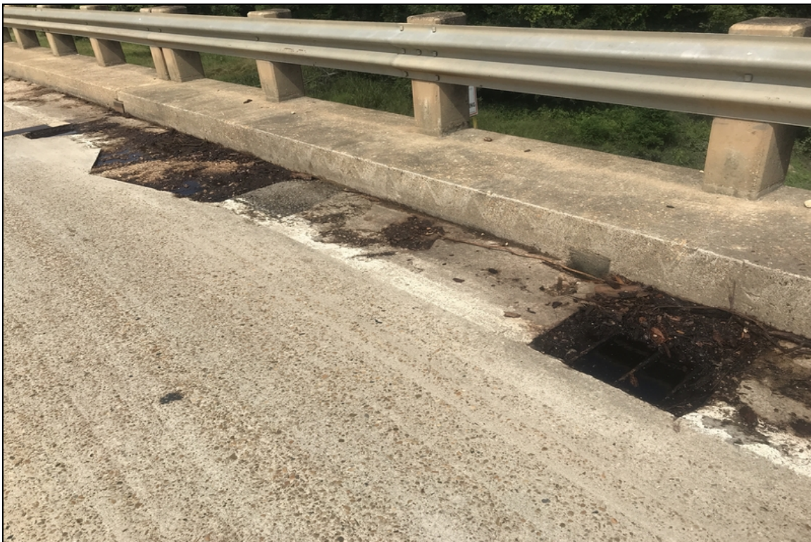
Span 25 spalls with exposed rebar in gutter line.
