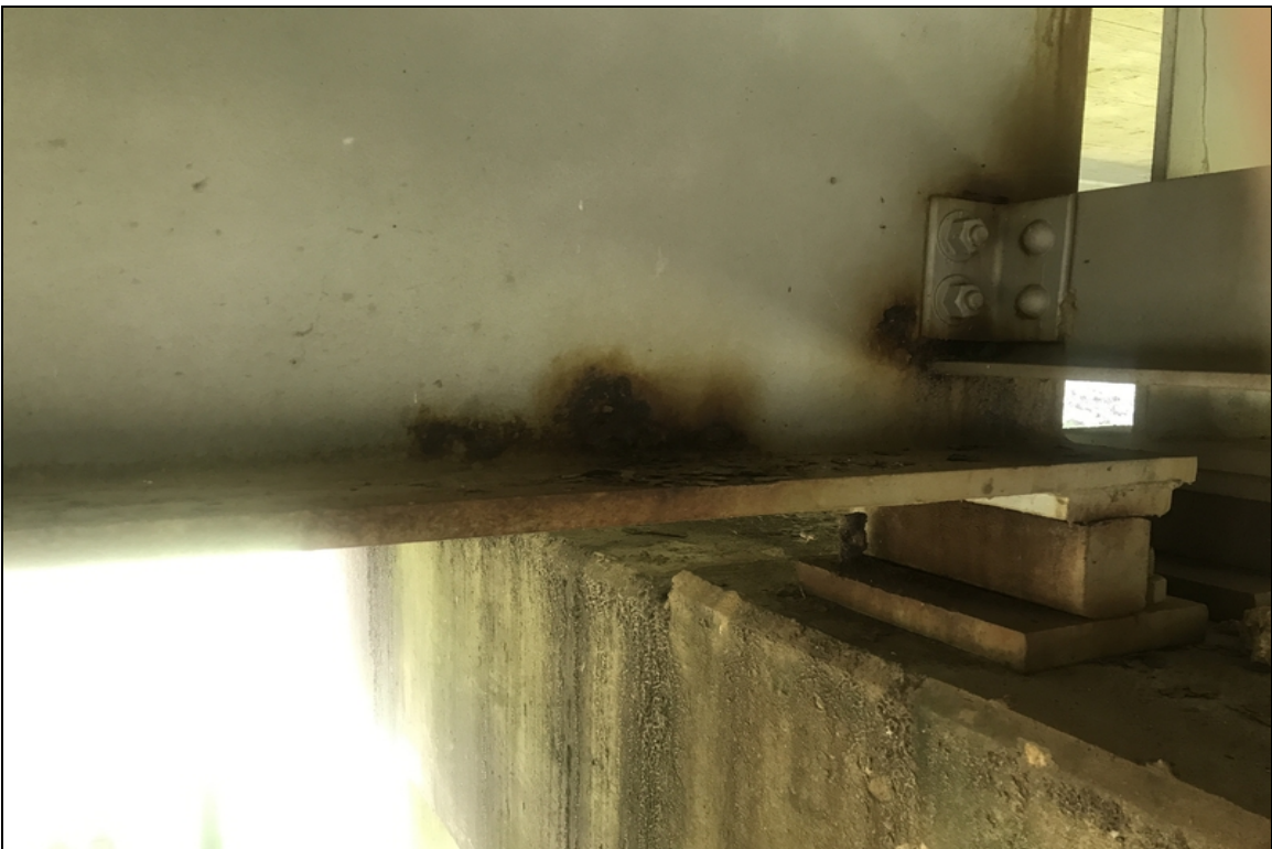
Span 27 beam 2 bent 28 flaking rust
