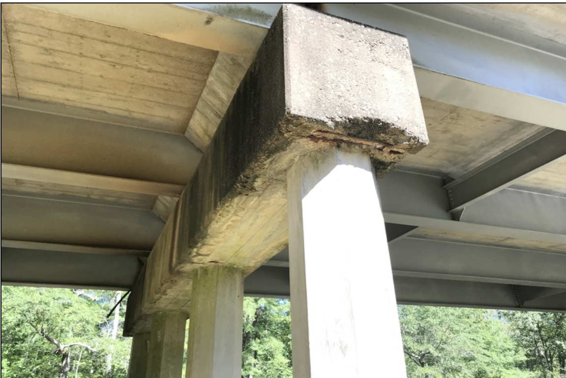
Bent 15 cap spalled right side
