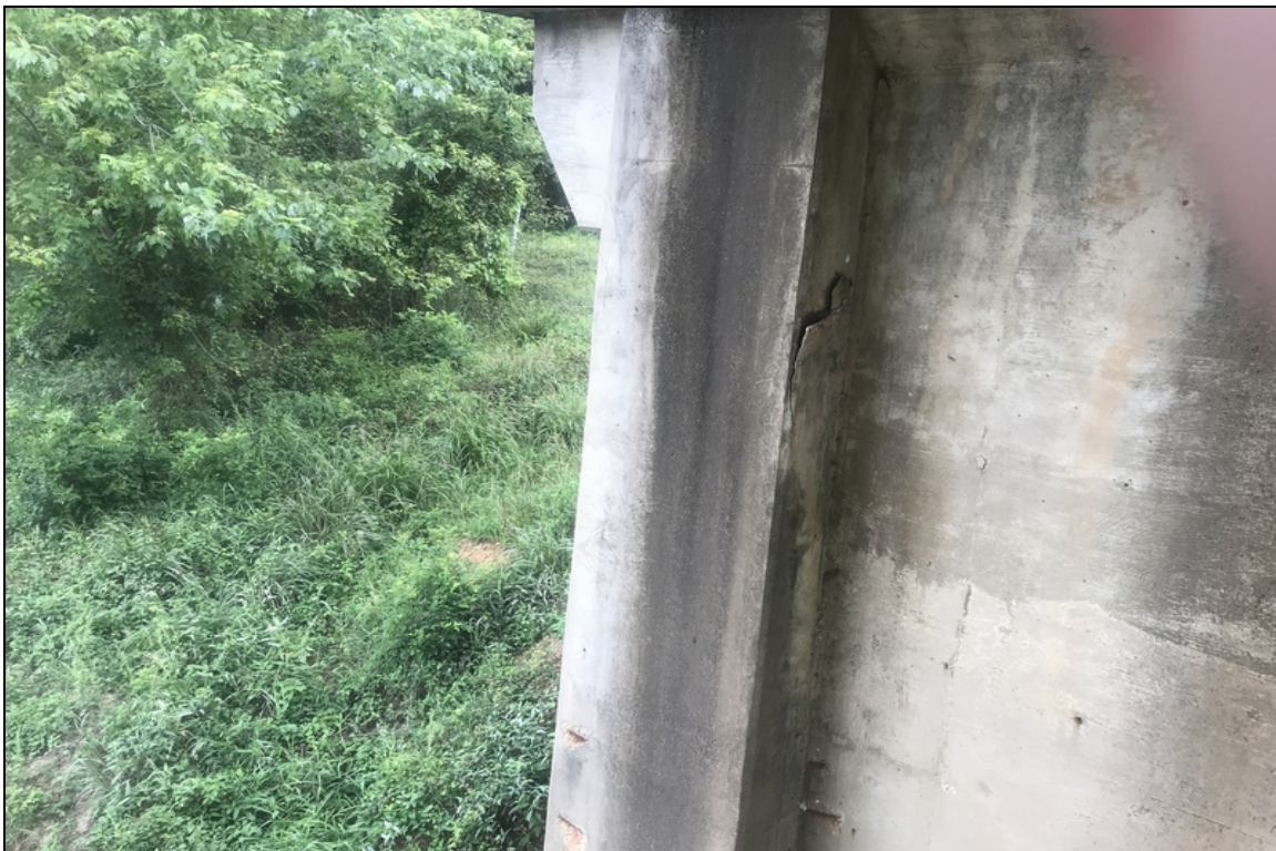
Pier 2 crack and delam with spall with exposed rebar
