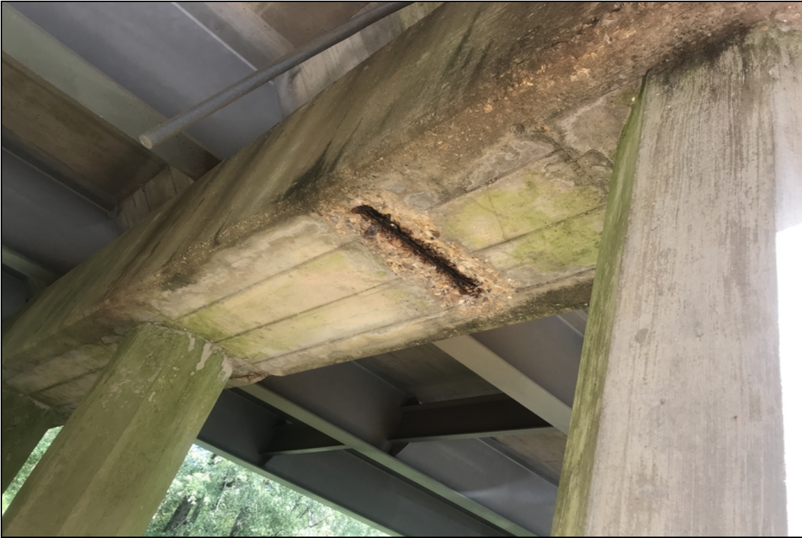
Bent 8 spall with exposed rebar, between piles 3-4.
