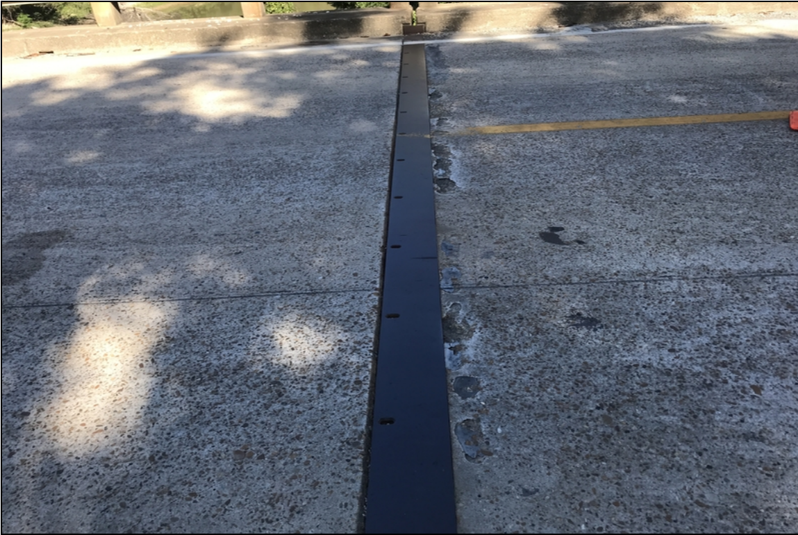
Bent 27 looking across @ joint between spans 27 & 28. There is some minor spalls on the ahead side of the joint.
