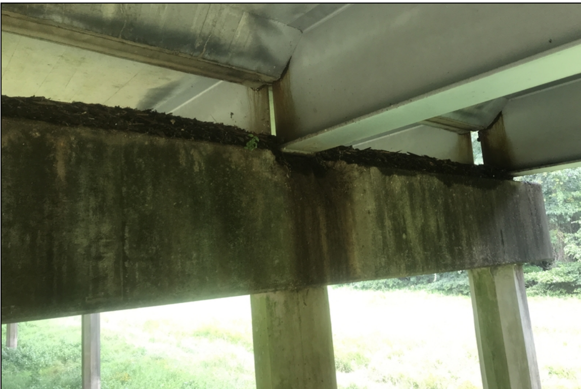
Bent33 cap spall
