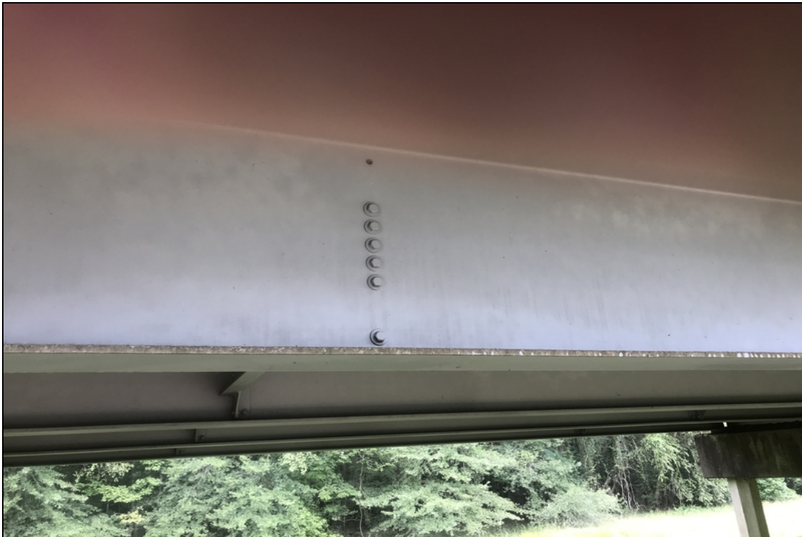
Span 41 beam 4 top bolt missing from diaphragm
