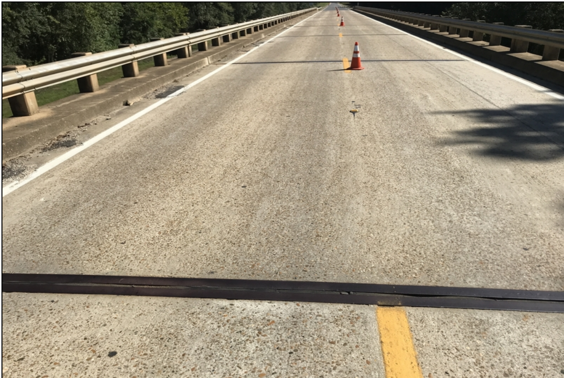
Span 40 looking ahead @ deck overview with some spalls in Lt. gutterline.
